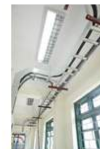
Elevator system and dynamic electric cables
